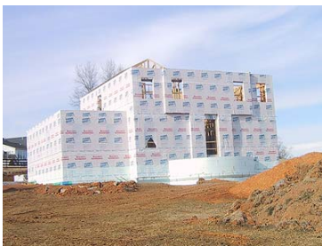
Construction of new homes is underway using the Health House® Guidelines.
